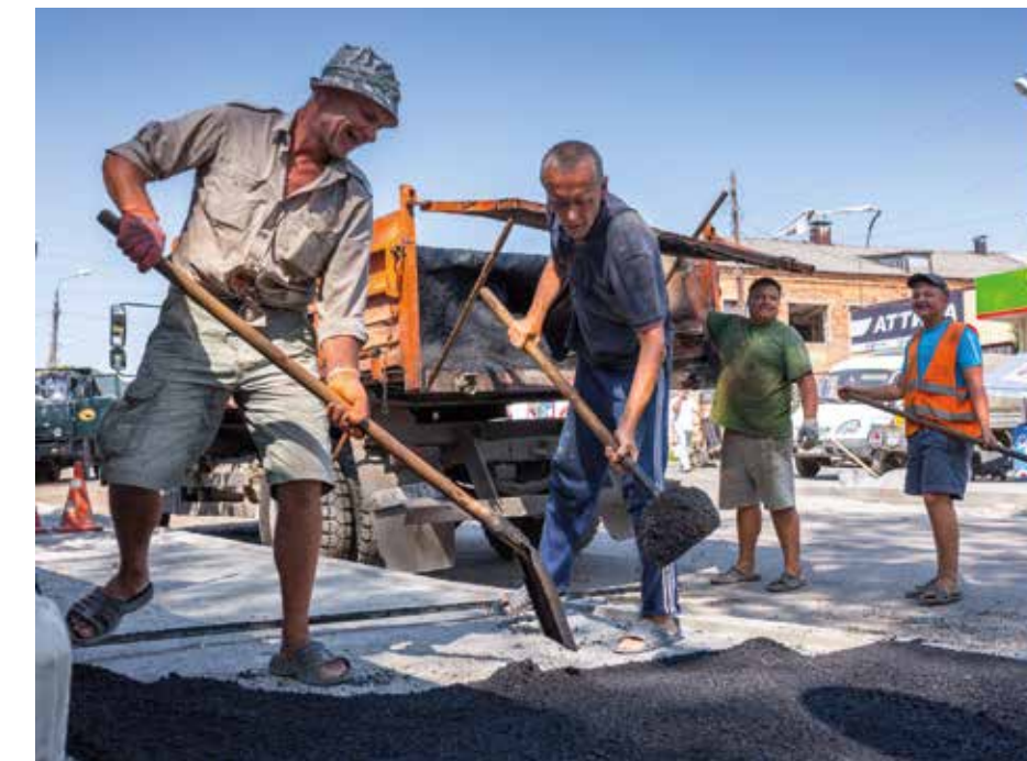
Road renovation in Merefa. August 2018
