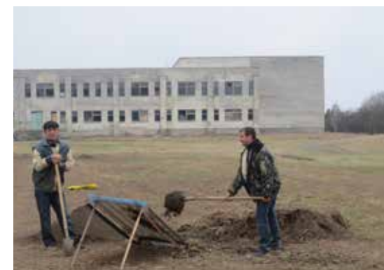
"Askania-Arena" renovation. March-September 2017
